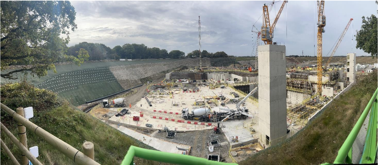
Figure 2.3: Construction Status of the Consented Scheme
